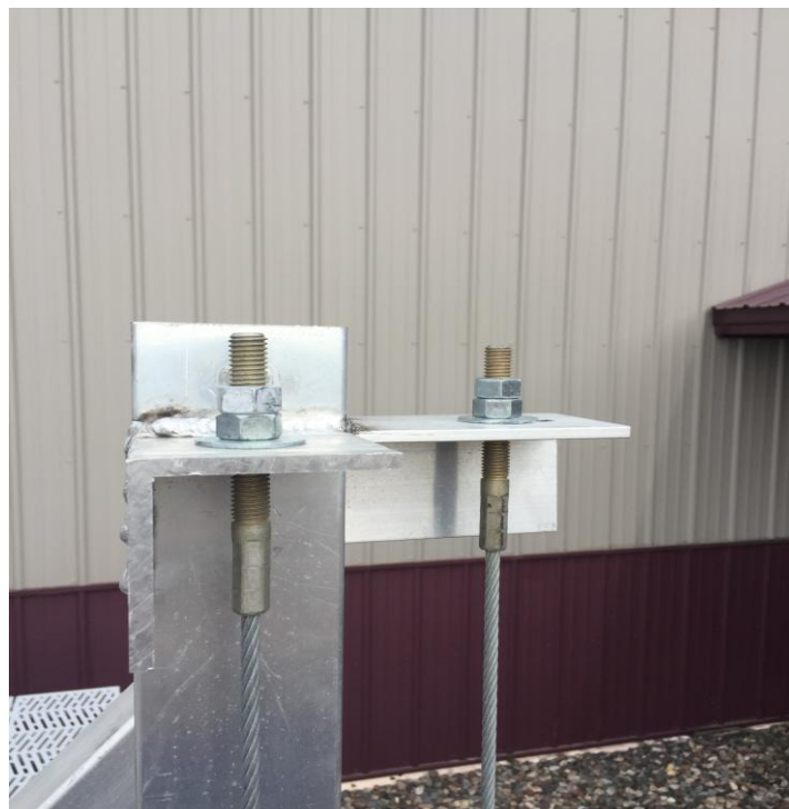
Notice - Nuts stacked to ensure no cable slip
