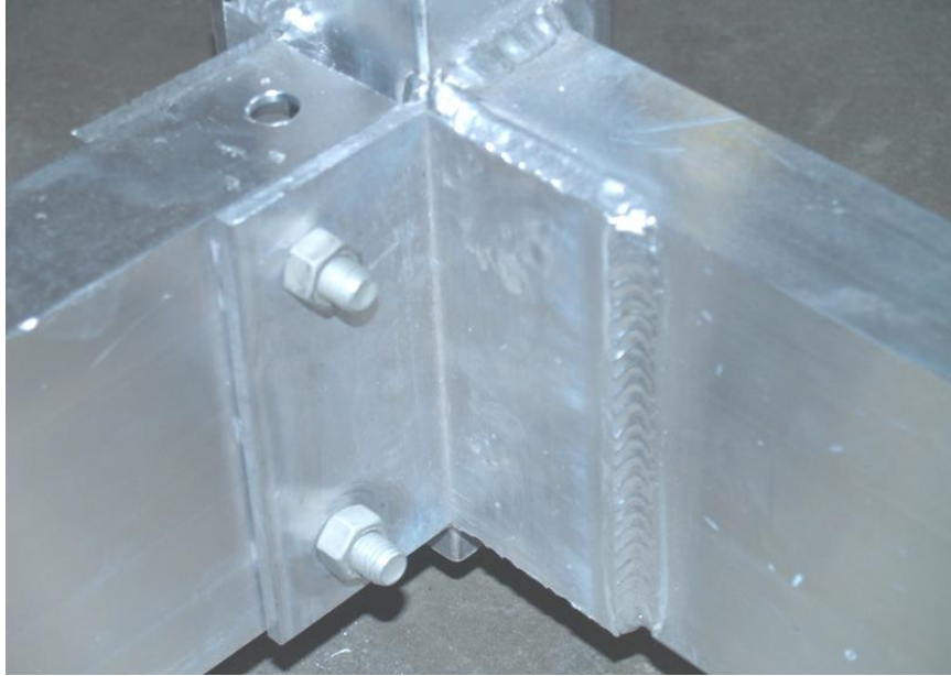
Close-up of frame cross members bolted to welded side frames.
